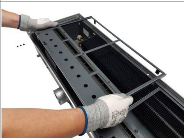
Fig. 9: Lift the baffle plate
