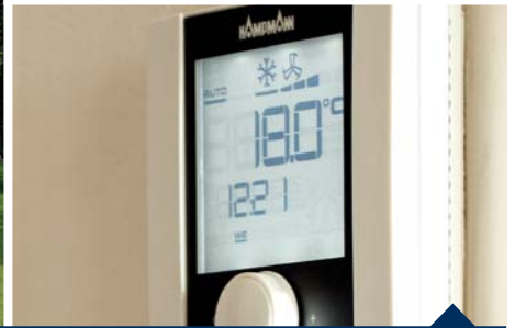
Venkon Fan Coil & KaControl Room Control Unit
